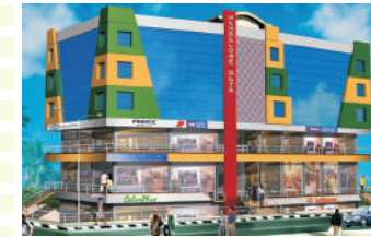
Mangalore Gate Kankanady, Mangalore (Completed)
